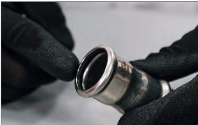
Controllo O-ring / Checking the sealing ring
